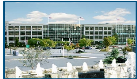
New and Rehab – Mixed Use/Office/Retail/ Medical
