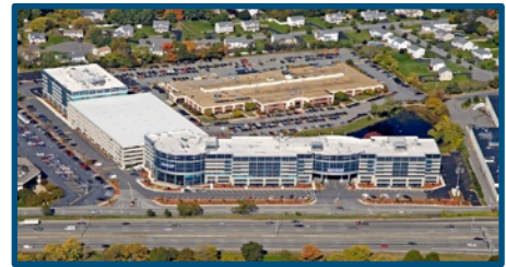
New Construction – Commercial Office
