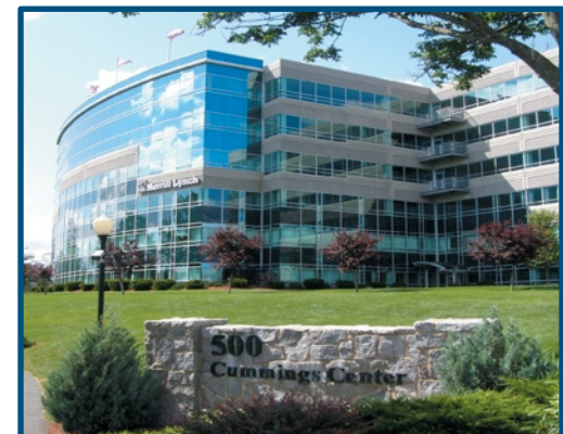
New Construction – Commercial Office
